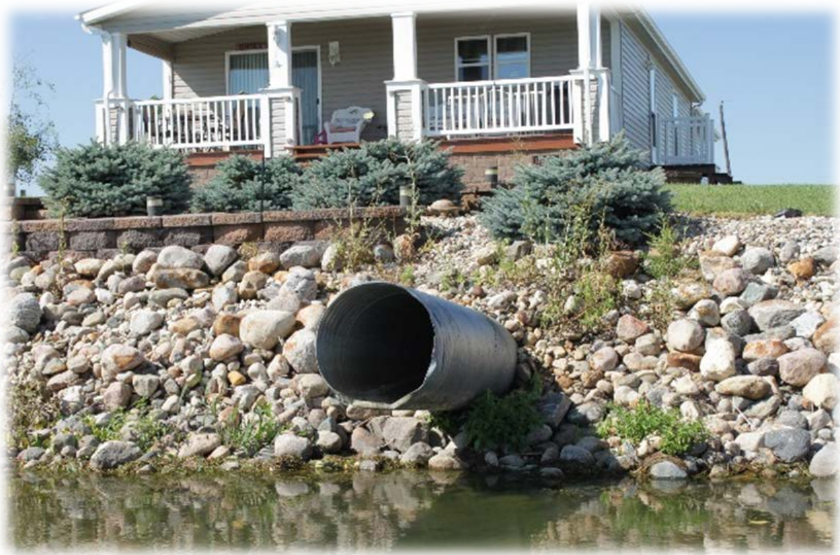
Figure 14. Drainage Culvert located in Block's Bay
