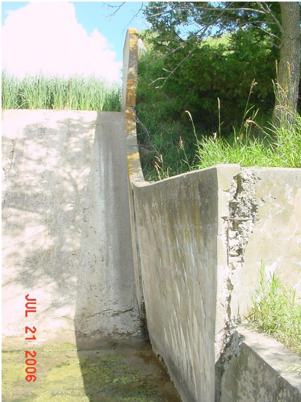
Figure 8. Pierpont Lake spillway structure (photo by Dennis Skadsen)
