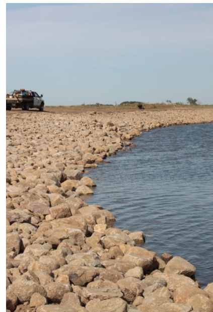
Figure 6. Amsden Dam after Stabilization
