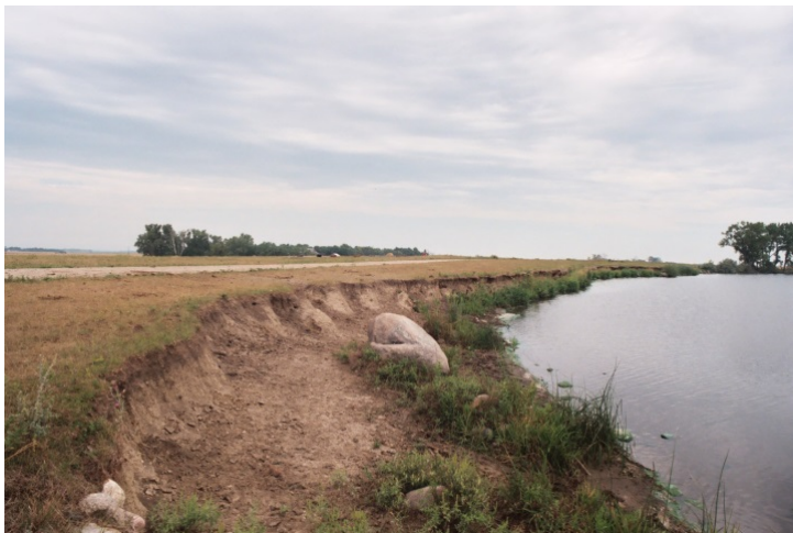
Figure 5. Amsden Dam before Stabilization
