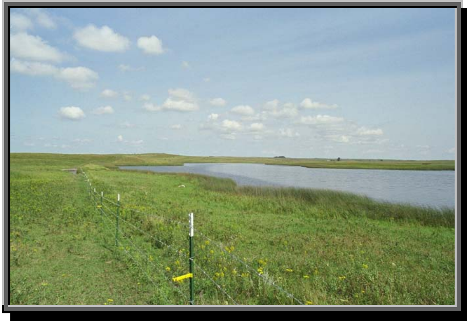
Figure 6. Buffer Fence Installed Along The Lake's Main Tributary.
